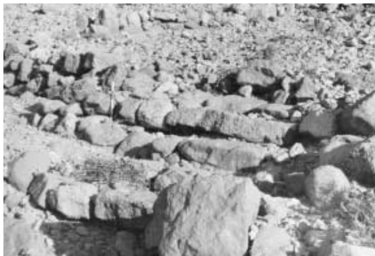
Fig. 62: Dams to restrain the streambeds
